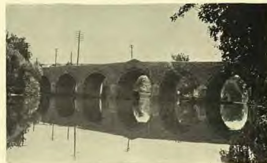
WITMER BRIDGE, BUILT IN 1800
