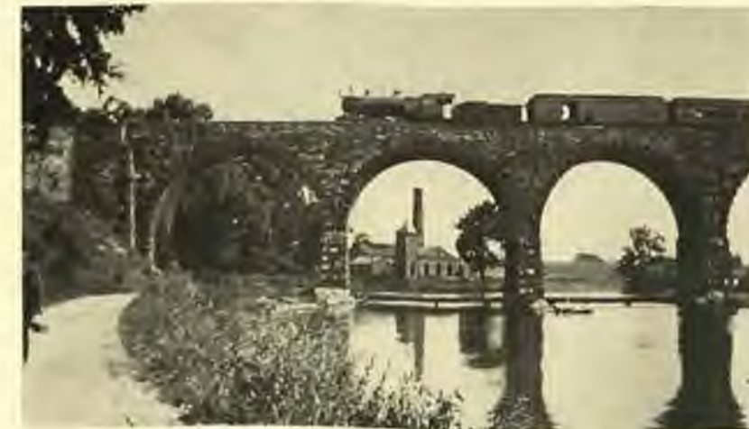
LANCASTER CITY WATER WORKS
